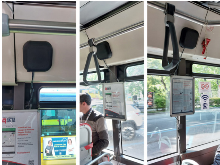
Figure 72: ETH's environmental sensors for air-quality monitoring system
